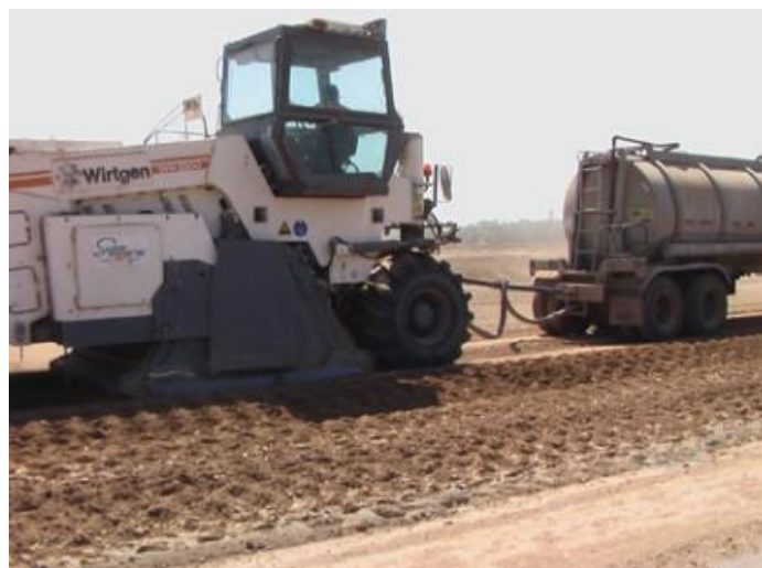
Figure 4. Mixing soil-cement for subgrade stabilization
